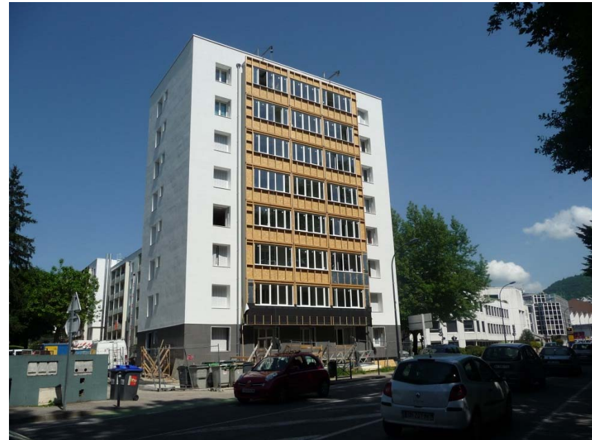
Voiron - During renovation Foto: E2ReBuild
