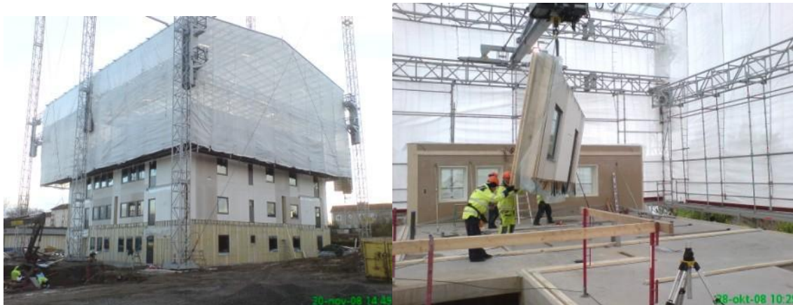
Figure 4. Weather protection. All assembly work takes place under protection against weather.
