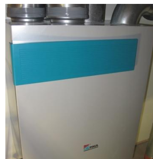
Figur 9: FTX-aggregat
